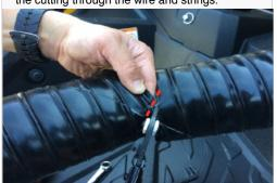
28. (Optional) Regular staples can be used to secure the ends of the strings to the duct.
